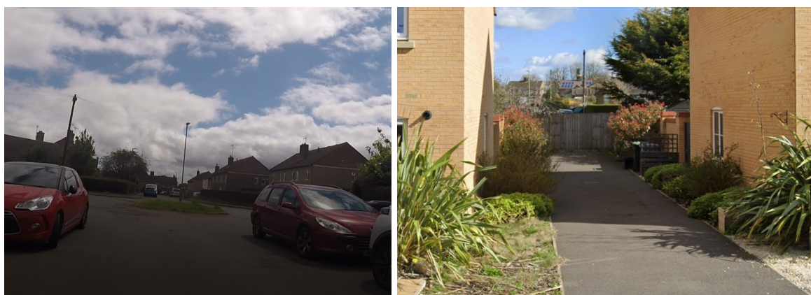
Figure 37 (left) - On street parking at mini roundabout
